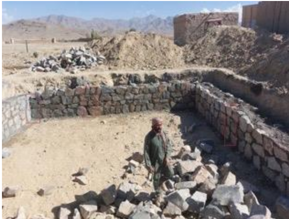
A water reservoir is constructed for the installation of a drip irrigation system in Logar Province.
