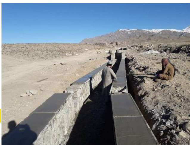
The Kanni Kulaw canal in Paktia Province is shown nearing completion.
