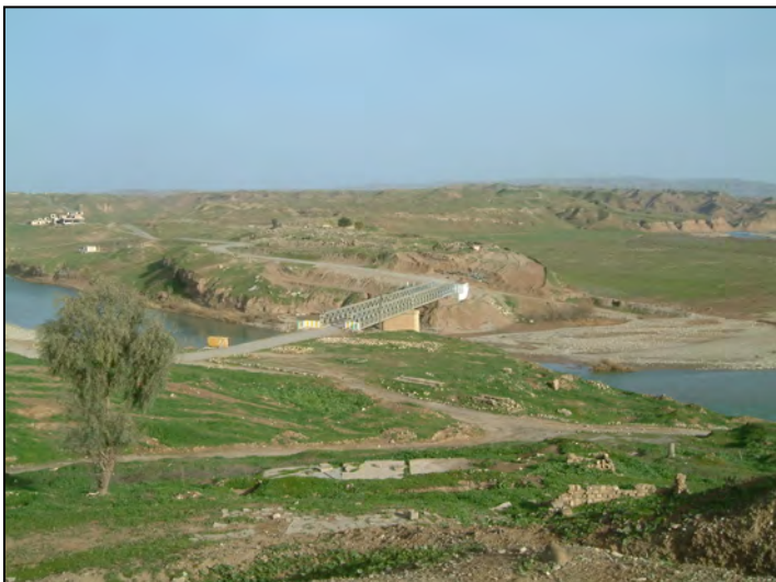
The repaired bridge crossing the Rokhana River in Qadir Karam. Minefields cover the area of land in the far right where one MAT is working.
